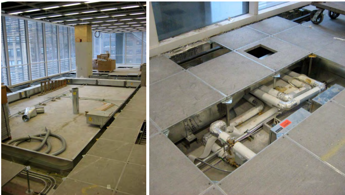
Figure 18. Images of the initial construction of the underfloor air distribution system. Copyright: LBNL.
