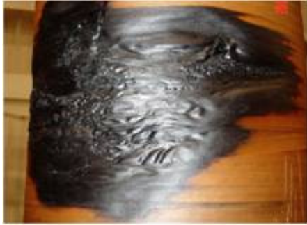
Fig. 3: Example of a current transformer with 6400 ppm C_2H_4 and no failure observed in service
